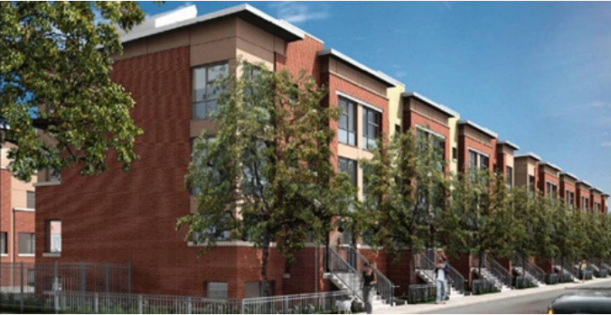
Social housing replacement units at 30 Regent Street, Toronto
