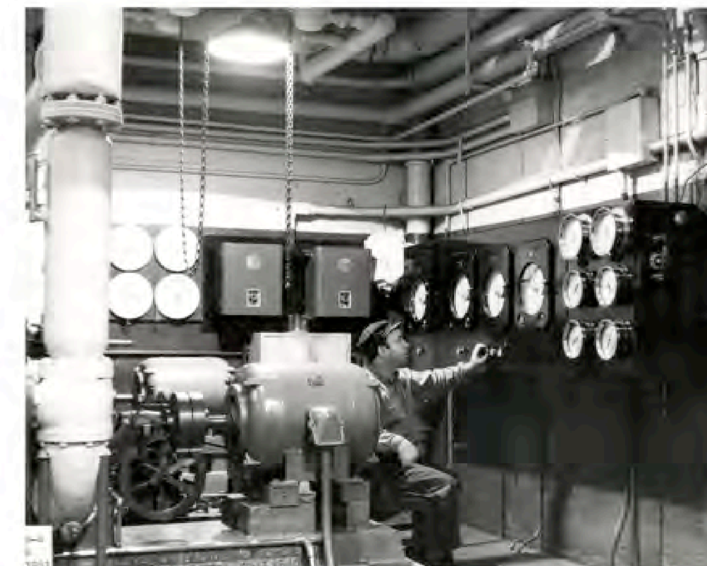
Engineer in Boiler Room, 1961
